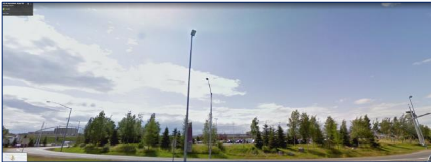
Figure 1: Example Street Lights Upgraded
