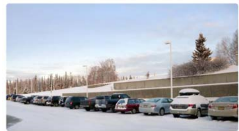
Safety is key during transitional seasons at each campus.
