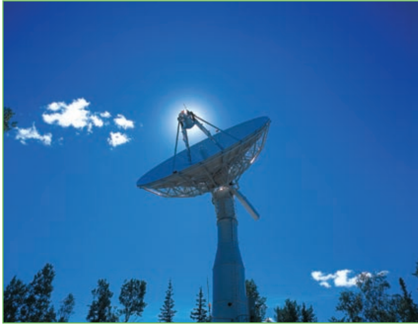
The Alaska SAR Facility's 11m parabolic dish collects data downlinks from multiple synthetic aperture radar satellites numerous times each day helping scientists at UAF and around the world view the earth's surface day or night, rain or shine.
