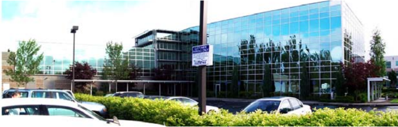
ACS Data Hosting Facility, Hillsboro, OR
