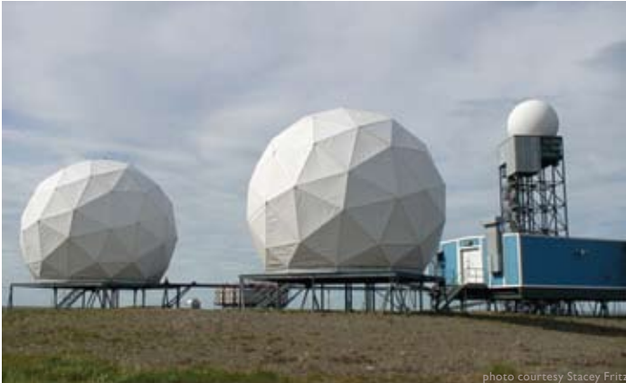
A typical DEW Line site.
