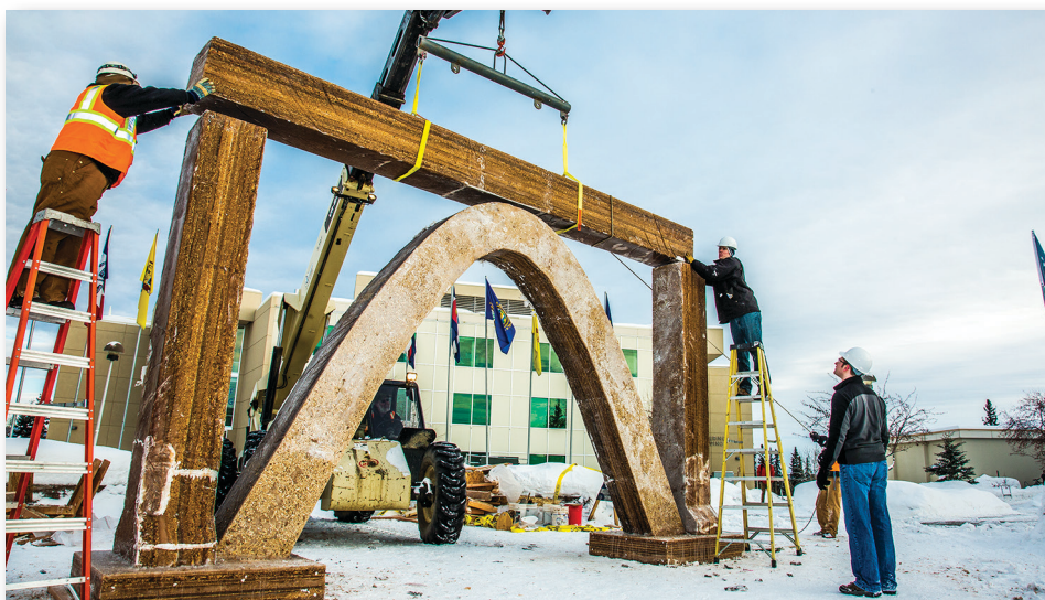
Engineering students Pat Brandon, on the ladder on the right, and Andy Chamberlain, on the ground, and volunteers from GHEMM Company stabilize the top piece of the 2013 ice arch as it is placed in Cornerstone Plaza on the Fairbanks campus. Students this year built the structure out of pyekrete, a mixture of ice and sawdust, which is eight to 10 times stronger than concrete.
