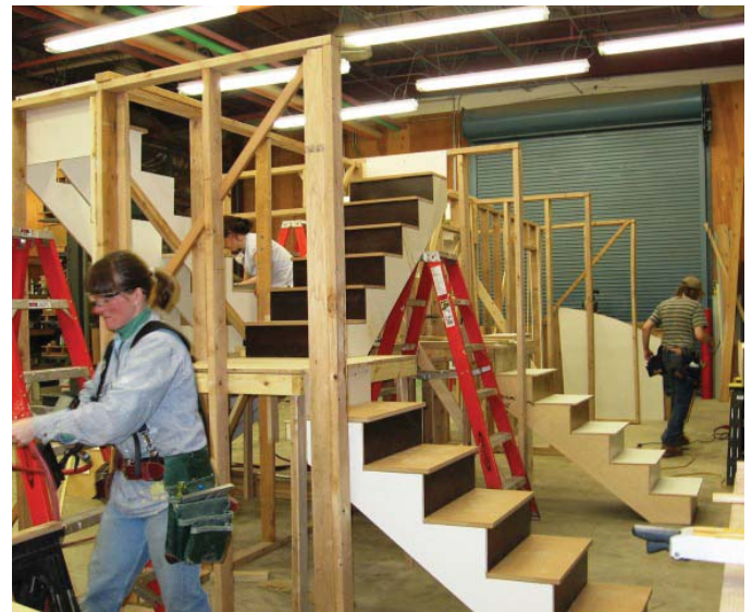
Photo 3.2 Stair Construction at TEC
