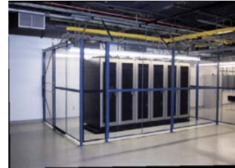
Installed Equipment Racks with Security Enclosure
