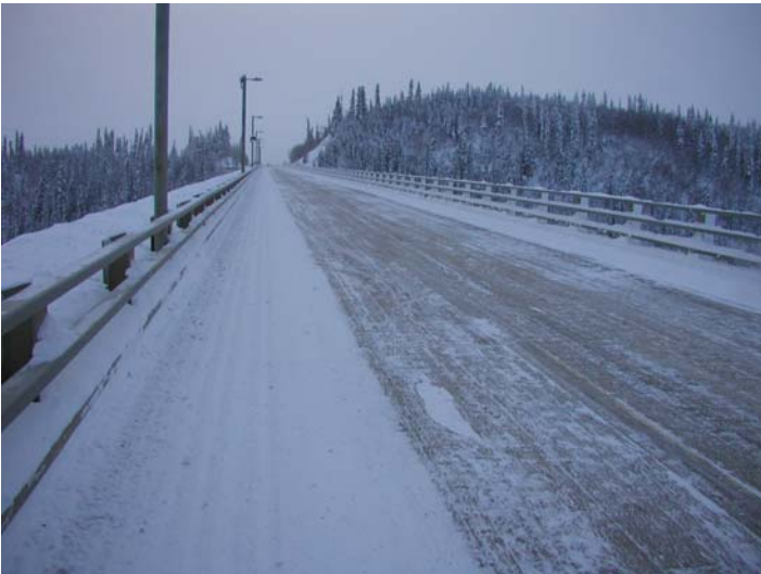
Figure 2. Yukon River Bridge in Winter
