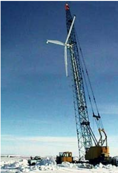
Erection of wind turbine at Kotzebue Electric Association.
