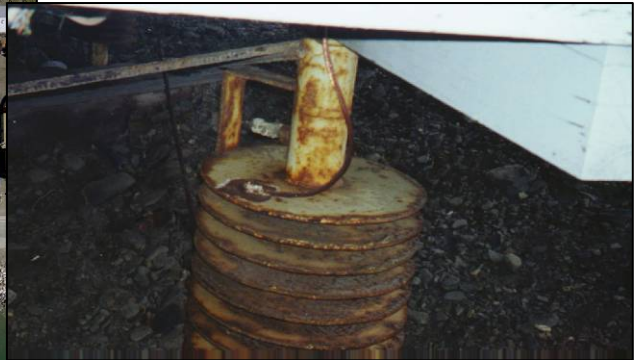
Library pilings in 2000
