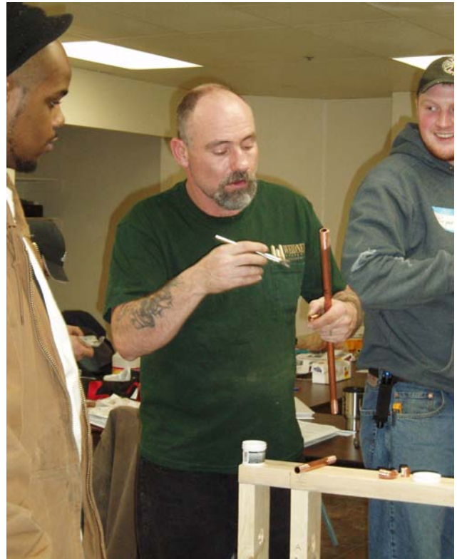
Participant Gary Snowball practices placing flux on copper piping.
